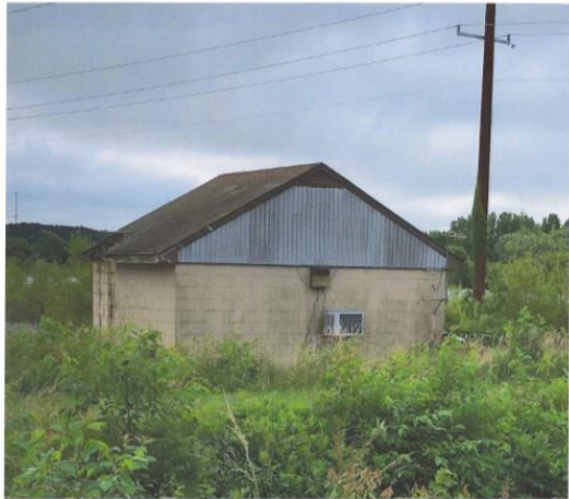
Building 7: On Pond. 20' X 13' 8" plus 6' X 20" overhang over water.
