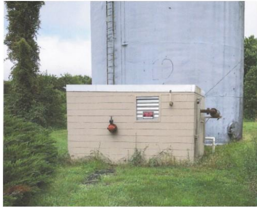
Building 2: Near water tank. 16' X 13' 6" plus 6' 8" extension connecting to water tank.
