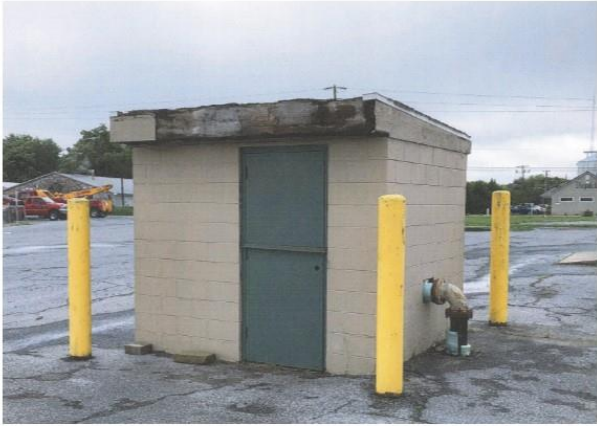
Building 1: Near front of property 10' X 8' concrete block
