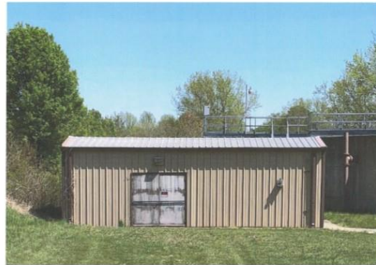
Building 4: Near concrete digester. 39' X 20' 1"
